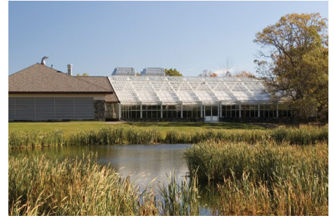
NEB's unique wastewater treatment facility treats the campus' wastewater for groundwater recharge.
